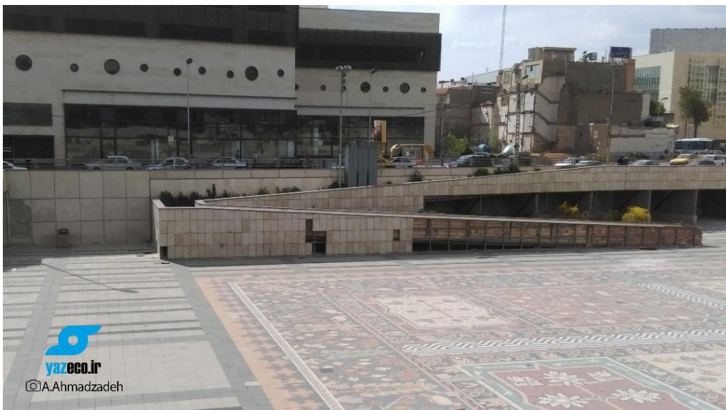
Figure 3.5: Deterioration of Beheshti Square materials Sources: Yaz Echo. bit.ly/3Yw69VM (visited: February 19, 2023)
