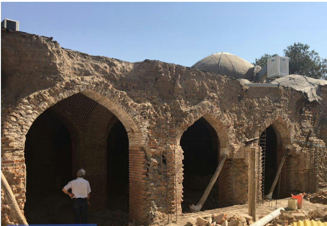
Figure 4.8: Karim Khan mosque before conservation Source: bit.ly/3SWw9Zk (visited: February 19, 2023)
